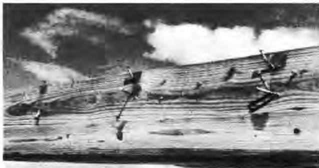
Figure 4.26. Toe Nailing Provides Limited Pull-Out Resistance
