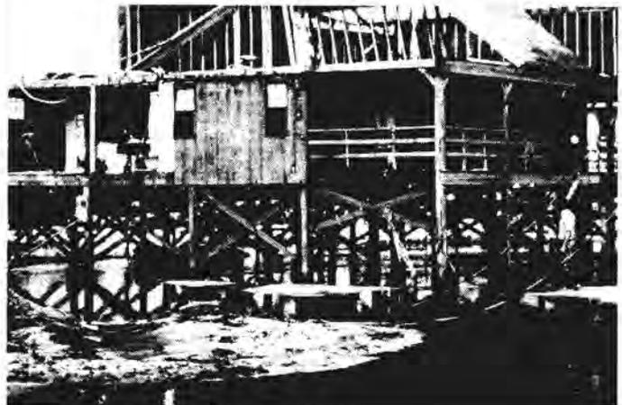
Figure 4.23. Diagonal Bracing
