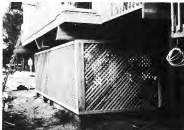
Figure 4.54. Breakaway Walls
